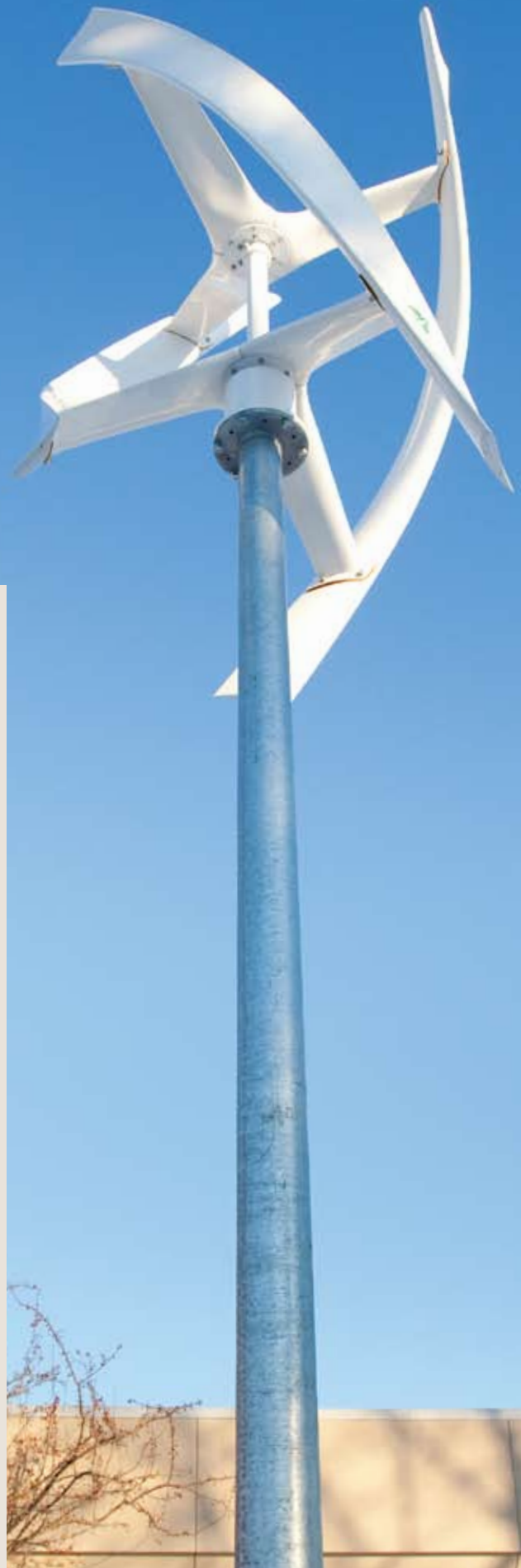
A 1.5 kW wind turbine stands outside IMPA's office building.
