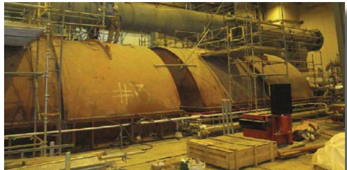
Turbine crossover pipe installation
