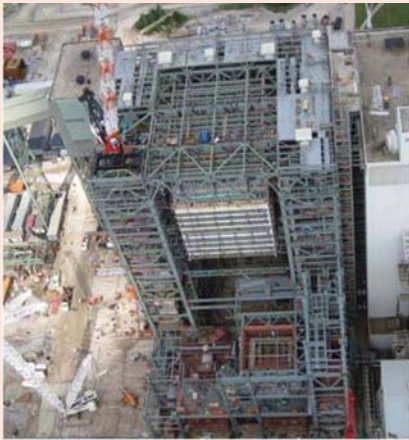
Trimble County Unit 2 Boiler Building
