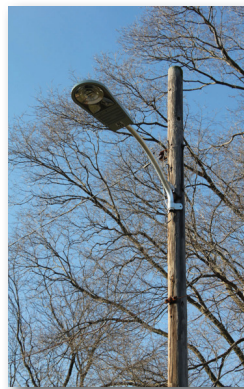
Greenfield's streetlights make a switch to energy efficient LED.
