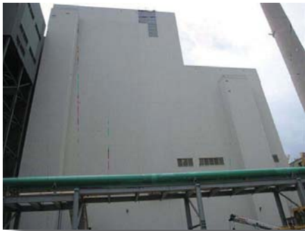
Trimble County Unit 2 is expected to be substantially complete this year.
