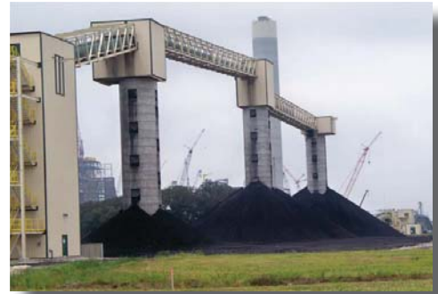
Lively Grove Mine coal stacking tubes at the Prairie State Energy Campus.
