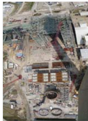
Overhead view of Trimble County Unit 2 construction
