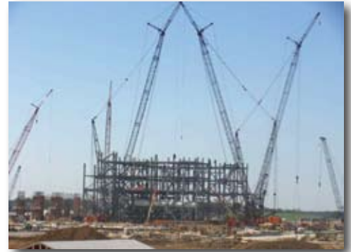
Prairie State STG Pedestal and Unit 1 Boiler Structural Steel - October 2008
