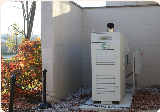
The IMPA microturbine is solely fueled by natural gas that is purchased from the retail market.
