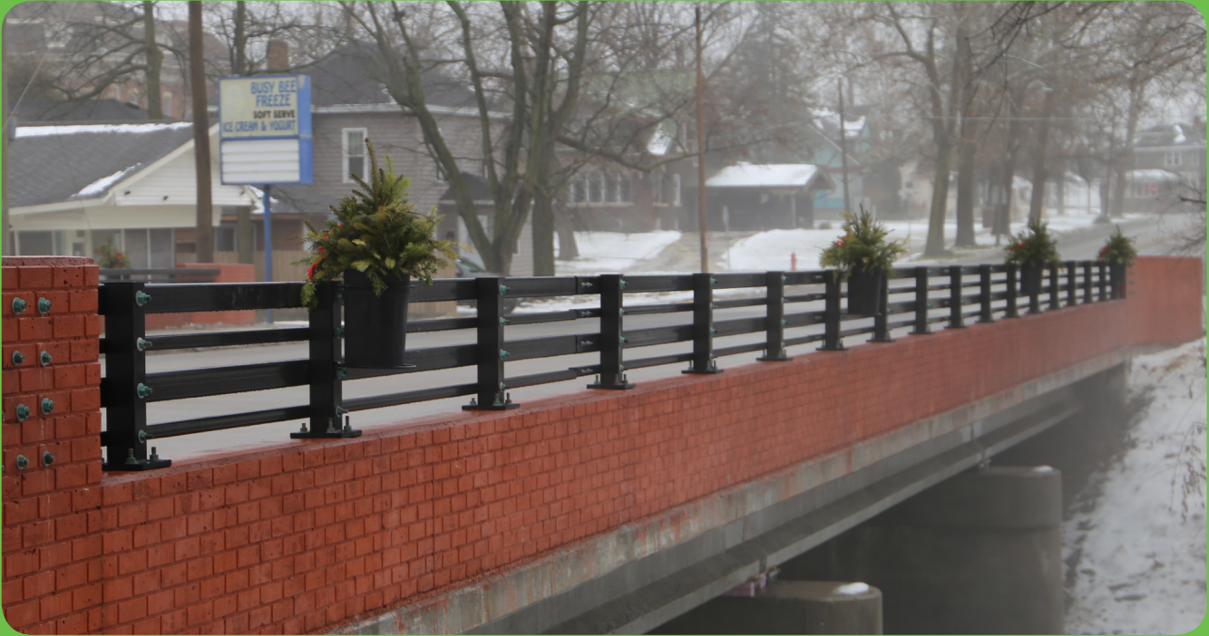
The Washington Street bridge is one of several projects the city has completed to improve the infrastructure of downtown Rensselaer.
