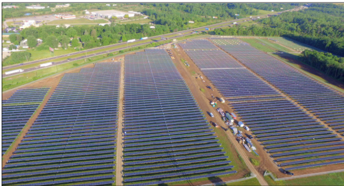
The photo above shows the progress of the 7.44 MW Richmond 2 Solar Park as of June 2018.
